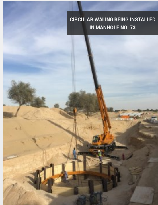
TYPICAL CIRCULAR SHORING SHAFT WITH MULTI LEVEL CIRCULAR WALINGS
