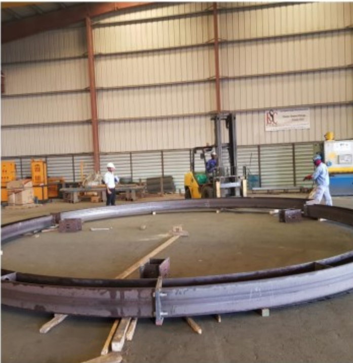
CIRCULAR WALING UNITS FABRICATION IN ESC YARD
