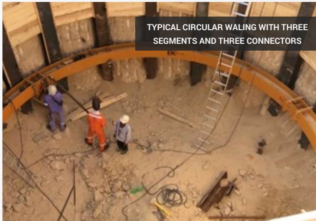
TYPICAL CIRCULAR SHORING SHAFT WITH MULTI LEVEL CIRCULAR WALINGS
