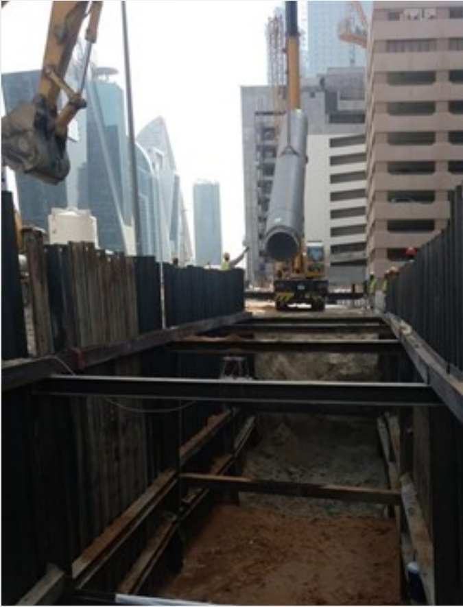
ESC TRENCH SHEETS INSTALLED AMIDST BUSY STREET IN DUBAI DOWN TOWN AREA FOR NEW PIPE LAYING WORKS
